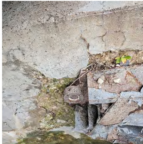
North Trunnion Condition, Delamination & Structural Deficiencies
