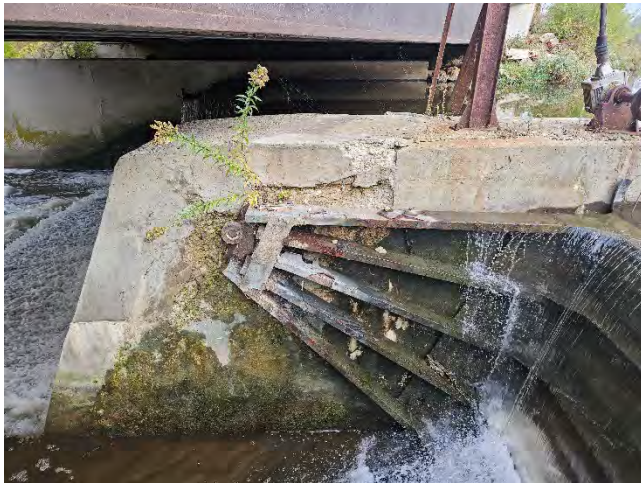
North Trunnion Condition, Delamination & Structural Deficiencies
