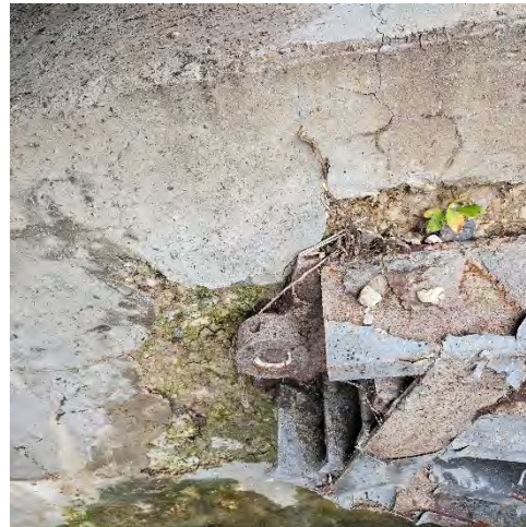
North Trunnion Condition, Delamination & Structural Deficiencies
