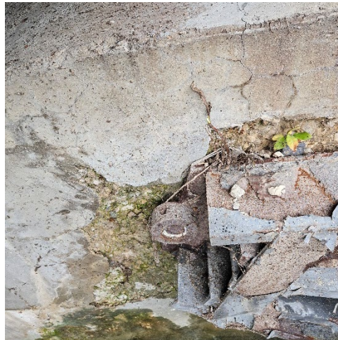
North Trunnion Condition, Delamination & Structural Deficiencies
