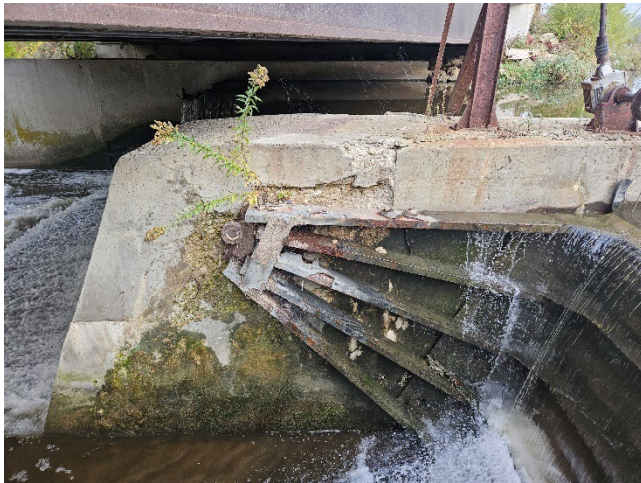
North Trunnion Condition, Delamination & Structural Deficiencies
