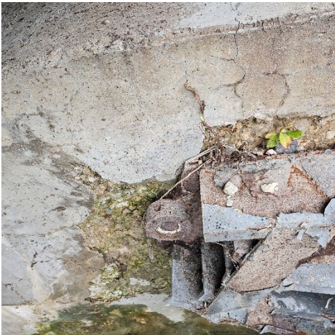
North Trunnion Condition, Delamination & Structural Deficiencies
