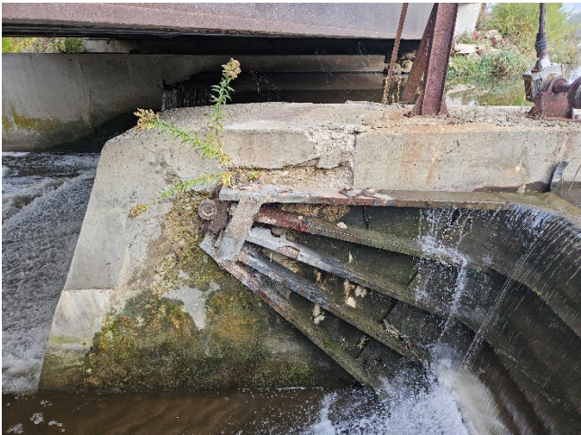
North Trunnion Condition, Delamination & Structural Deficiencies
